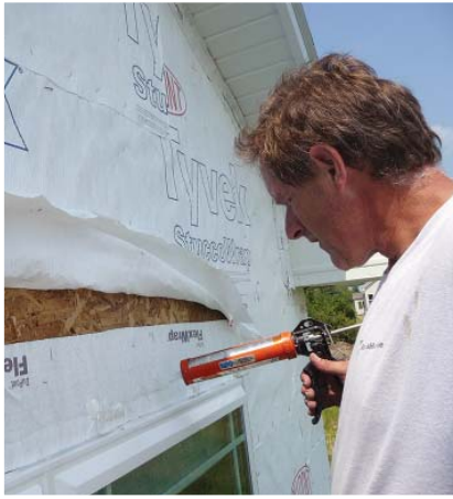
Figure 3. To limit water and air infiltration, the author applies a bed of sealant to the flashing tape above the window (above), then installs the metal cap flashing (right).
