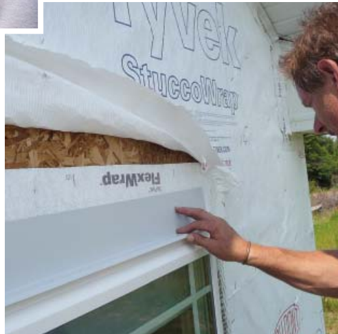
Figure 3. To limit water and air infiltration, the author applies a bed of sealant to the flashing tape above the window (above), then installs the metal cap flashing (right).
