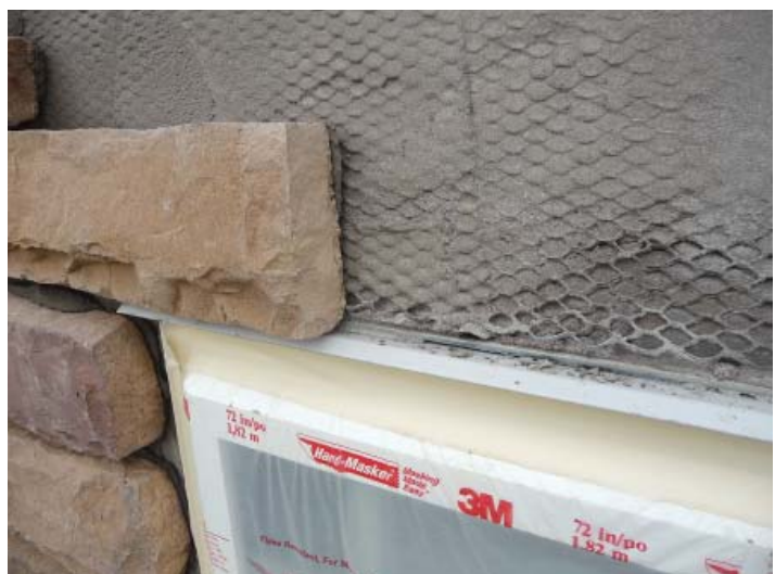
Figure 6. Like stucco, manufactured-stone veneer is applied over a base coat of mortar (left). The cap flashing (above) is sized to match the thickness of the stone veneer, to ensure that water is diverted to the surface.
