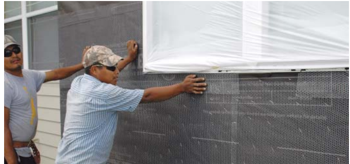
Figure 5. Crew members install a double layer of 60-minute grade D building paper on top of the StuccoWrap (above). The paper laps over a metal weep to allow for drainage at the base of the wall (above right). Galvanized metal lath (right) is then installed over the building paper.
