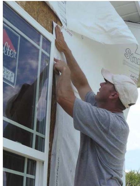
Figure 2. A sill pan fashioned from FlexWrap (far left), installed on top of the StuccoWrap, protects the rough window opening. The window is reinstalled with the nailing flanges set in sealant, then taped to the StuccoWrap (left).
