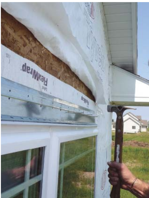
Figure 4. A metal weep screed above the window allows water to drain out from behind the cladding and mortar base coat (left). Metal J-mold is applied underneath the window (above left) and at the jambs (above right); flexible sealant is used to fill the joints between the J-mold and the window.
