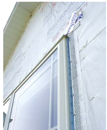
Figure 4. A metal weep screed above the window allows water to drain out from behind the cladding and mortar base coat (left). Metal J-mold is applied underneath the window (above left) and at the jambs (above right); flexible sealant is used to fill the joints between the J-mold and the window.
